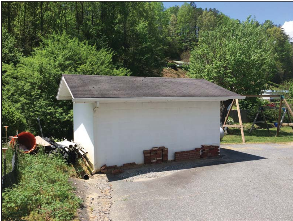
Photograph 9: East and south elevations of the block shed; looking west.
