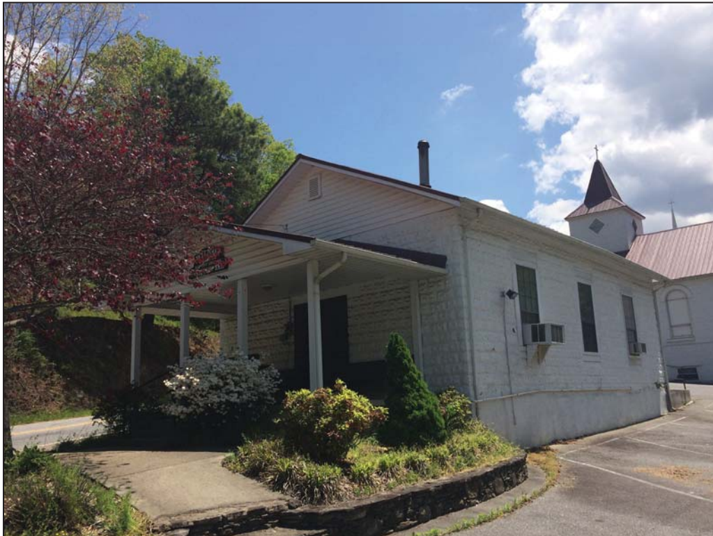
Photograph 1: North and west elevations of the original church; looking southeast.
