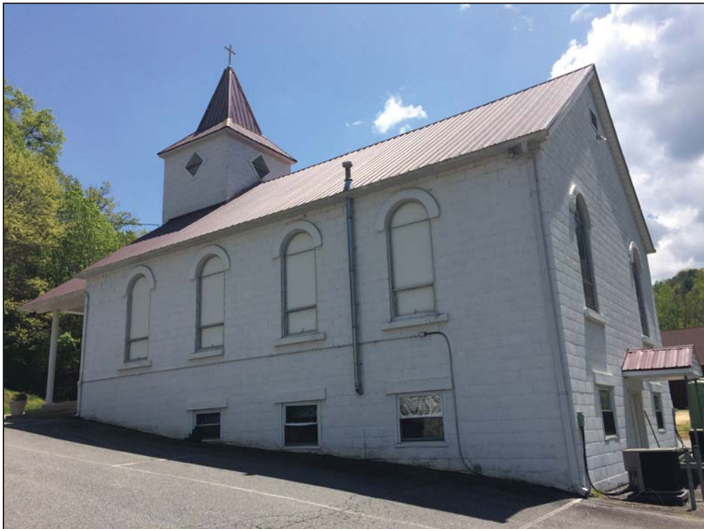
Photograph 7: North and west elevations of the c. 1947 church; looking southeast.
