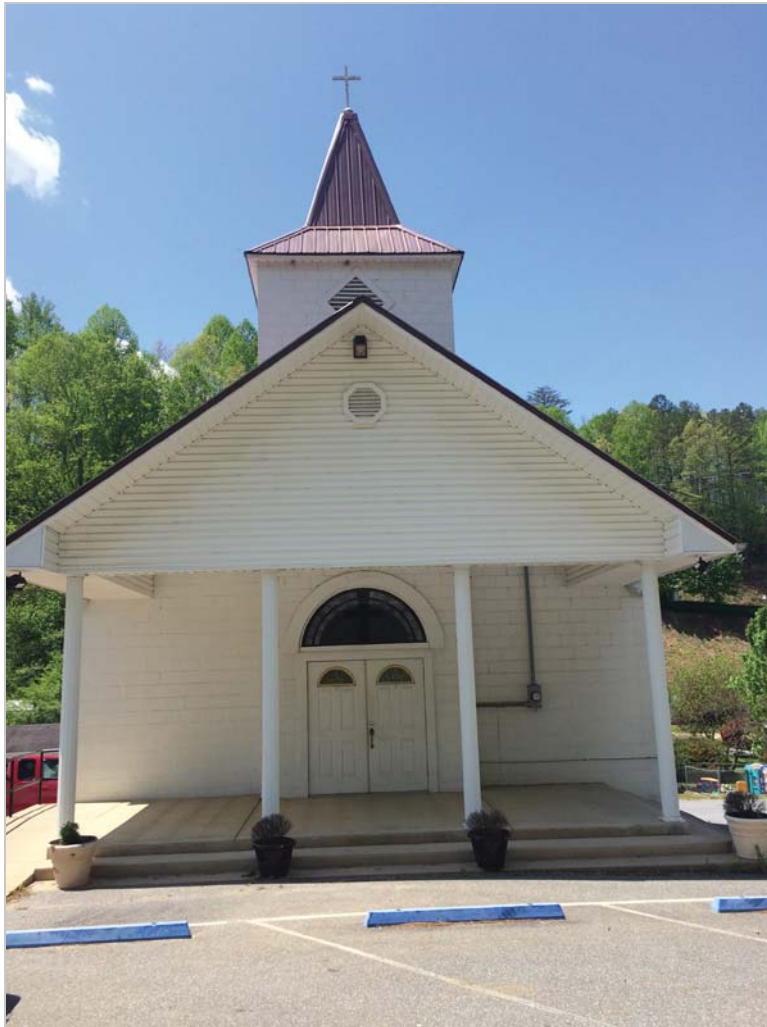
Photograph 6: East elevation of the c. 1947 church; looking west.
