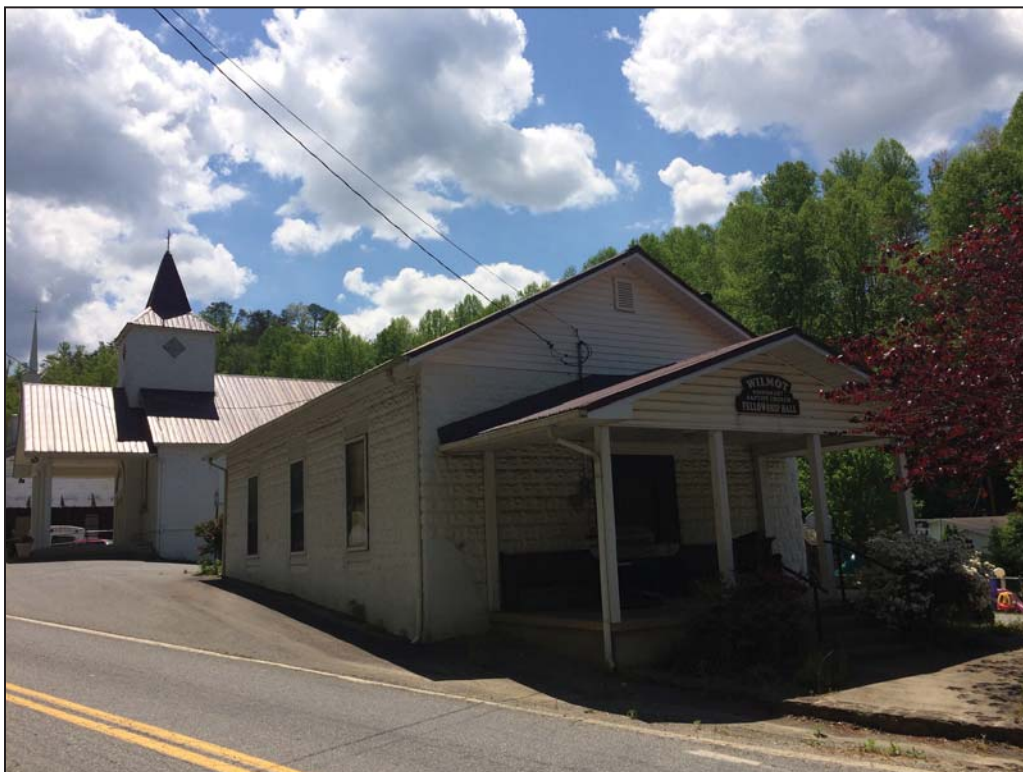
Photograph 2: North and east elevations of the original church; looking southwest.
