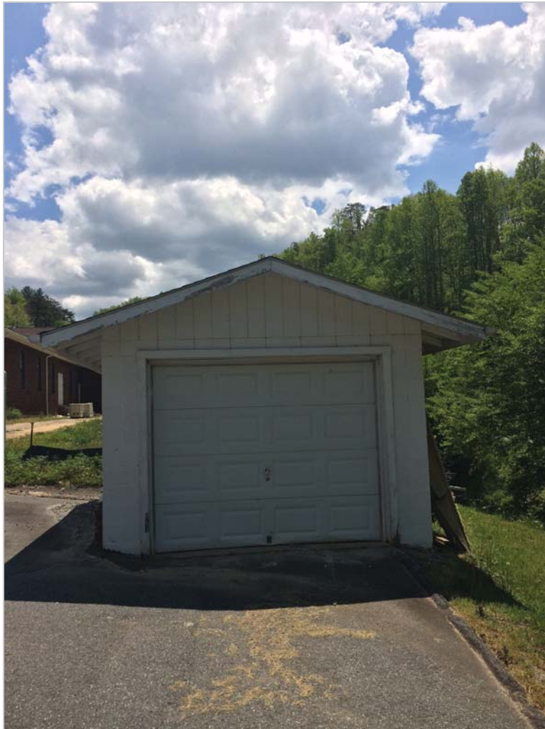
Photograph 10: North elevation of the block shed; looking south.
