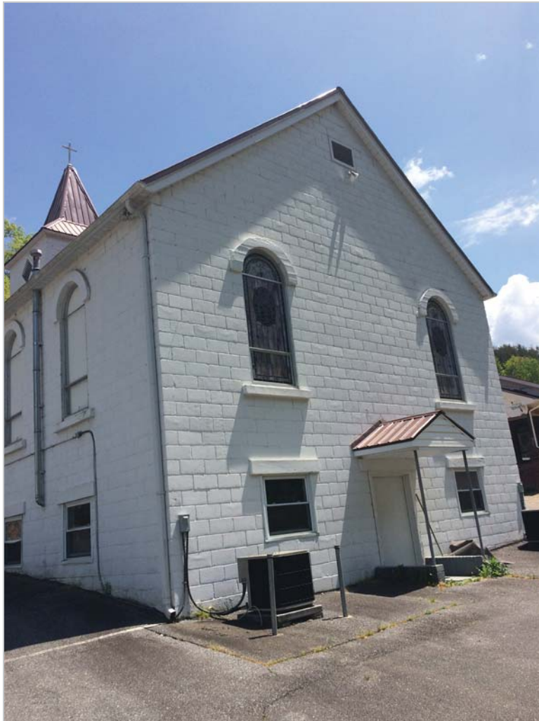
Photograph 8: West elevation of the c. 1947 church; looking southeast.
